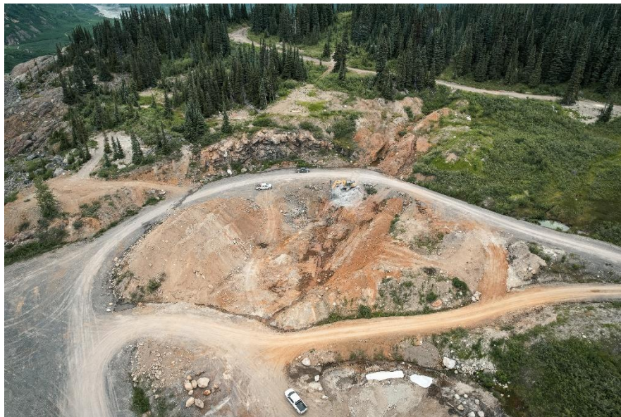
Figure 1 – Overview of Bend Vein zone and drilling prior to initial blast.
